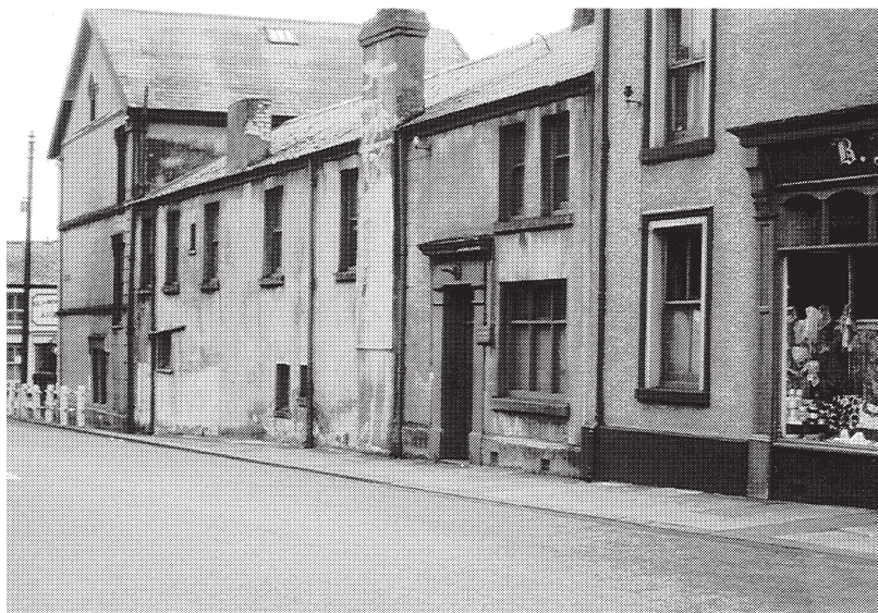
2, Brecon Road, Merthyr Tydfil
